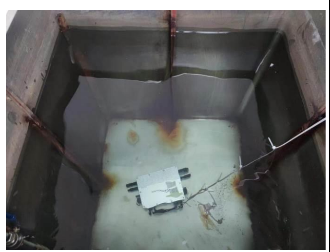
Photo 4 In the waterproof test
