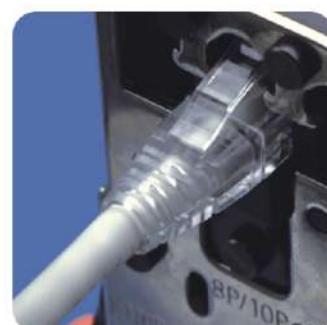
11.Place the RJ45 plug into a hand tool crimping die for compression.
