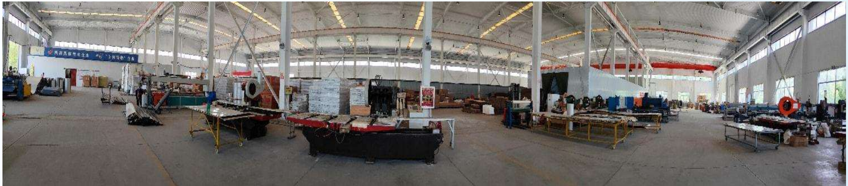
Solar Water Heaters Plant
