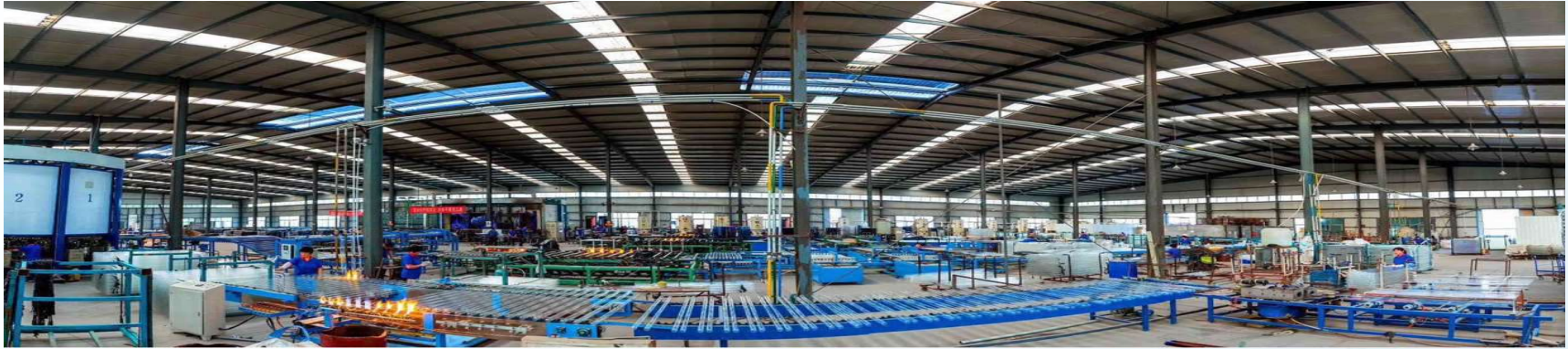
Solar Vacuum Tube Plant
