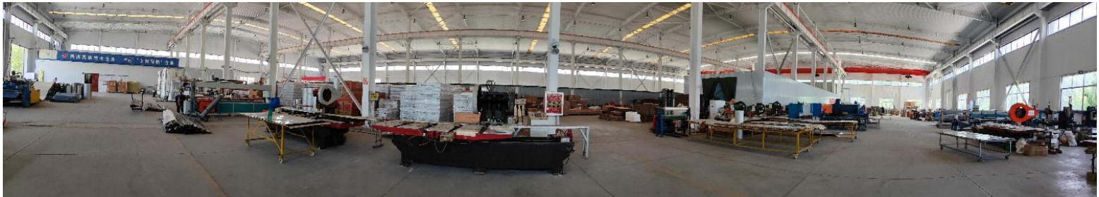
Solar Water Heaters Plant
