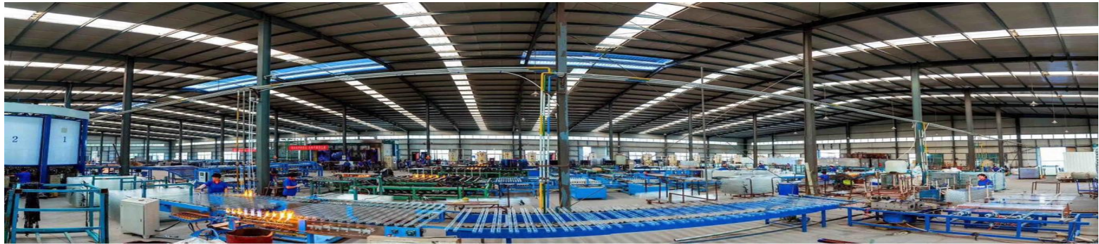
Solar Vacuum Tube Plant
